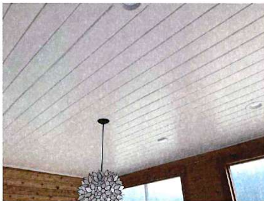
Enclosed Patio - Sun Room - NO HVAC
