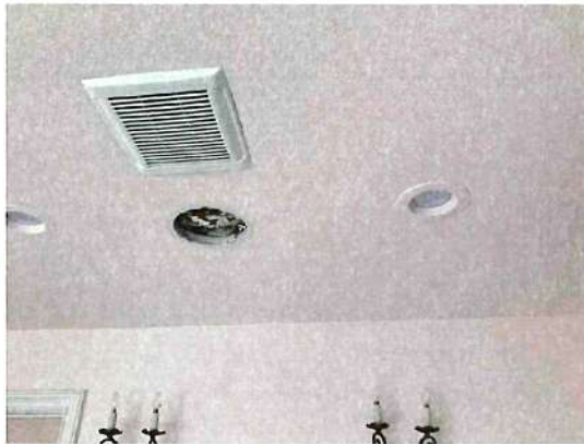
Bath - Hole In Ceiling - Speaker Not Installed
