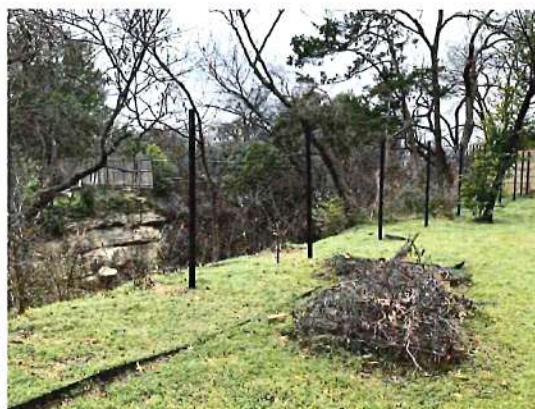
Missing Fence Section
